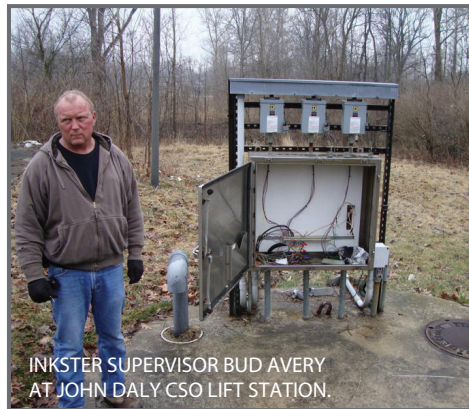
CSO LIFT STATION WITH BARNES SH SERIES
