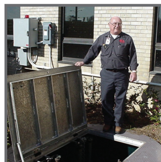
MARTY COLE AT WK NORTH MEDICAL CENTER LIFT STATION
