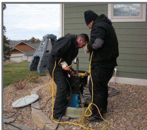
Precision Plumbing sent two installation technicians to the problematic site with a Barnes Replacement Core upgrade with the Omni Grind Plus grinder pump. The installation was fast and easy, and the upgraded station no longer suffers from failures or nuisance alarms.
