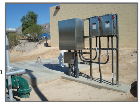
TOWN OF HAYDEN WASTE WATER TREATMENT PLANT
